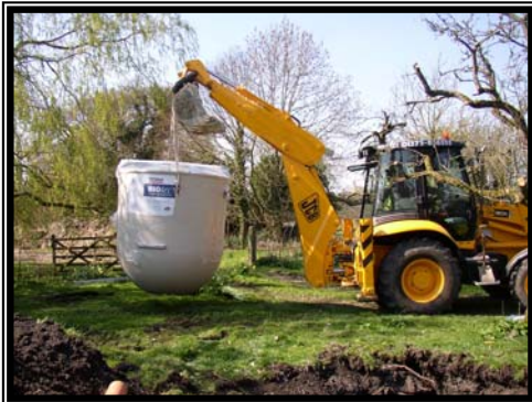
A SINGLE HOUSE, 6 PERSON TREATMENT PLANT INSTALLATION
